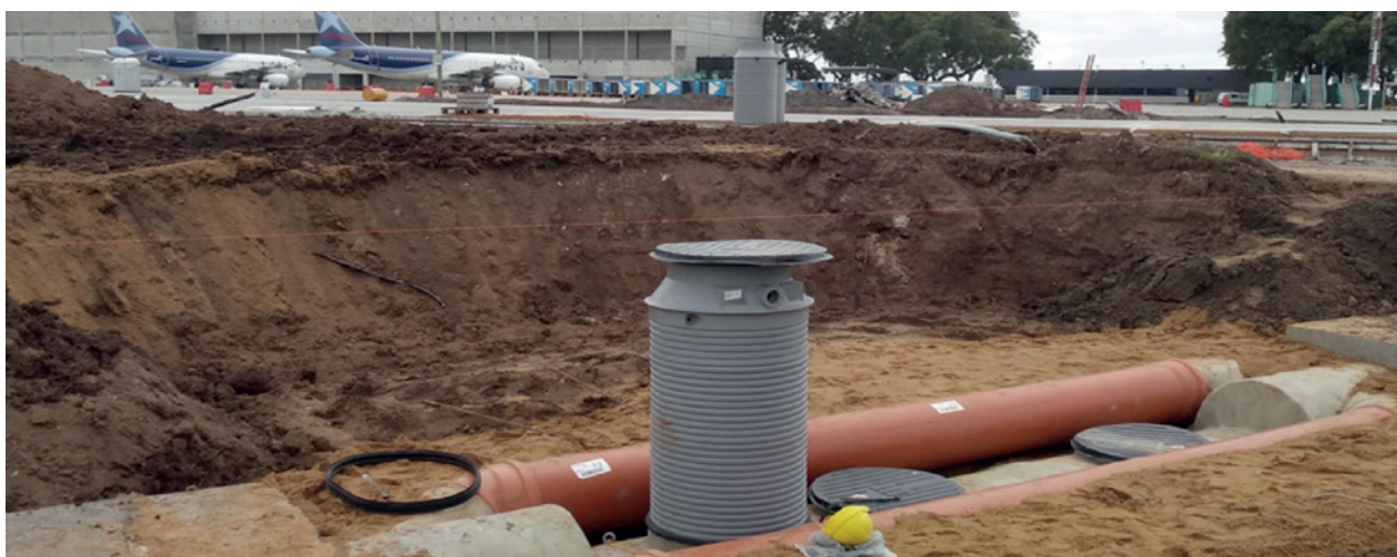
Arrival of the separator on site.
