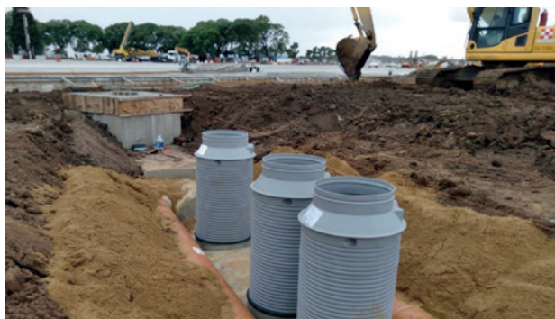
The separator being covered and final installation of the 3 access chambers
