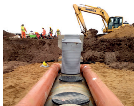
Perspective of the separator and bypass pipes.
