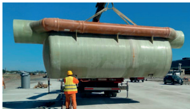
Arrival of the separator on site and preparation for descent into the excavation area.
