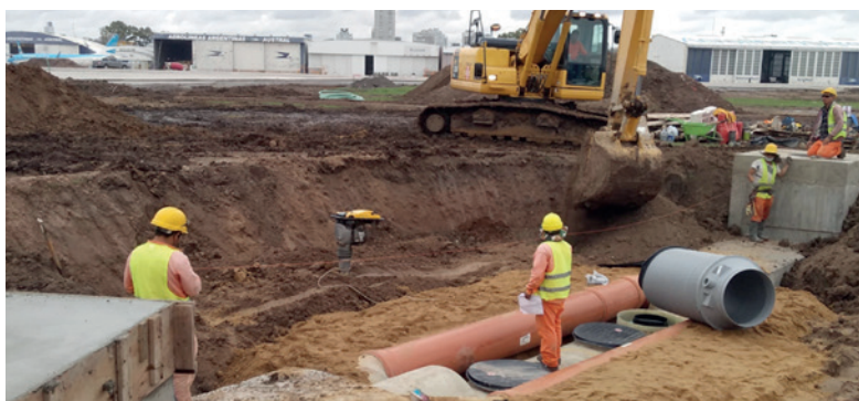
Separator installation work in the excavation area.
