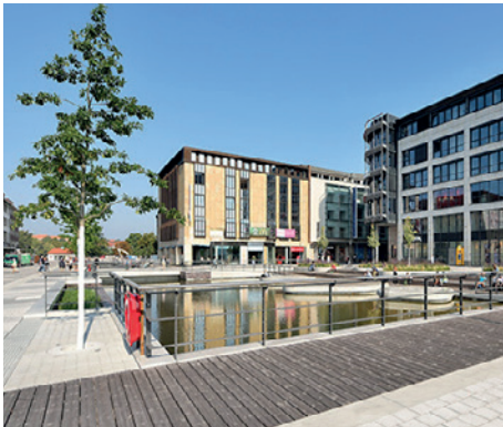
The south basin of Kiel's city centre
