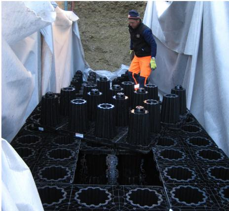
Building in existing structures, an excavation pit with the first layer of ACO Stormbrixx basic elements
