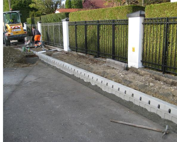
ACO Kerbdrain channel includes two functions - linear drainage and curb - in one component
