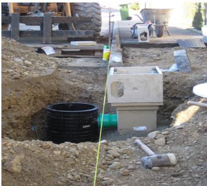
Sump unit of the KerbDrain channel in combination with the Combipoint road gully
