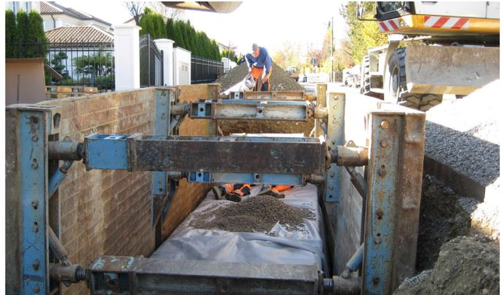
Excavation pit with a civil engineering formwork, due to its modularity the infiltration tank can be easily installed
