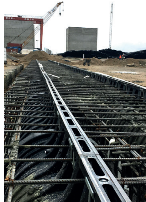
Main line installed phase 1
