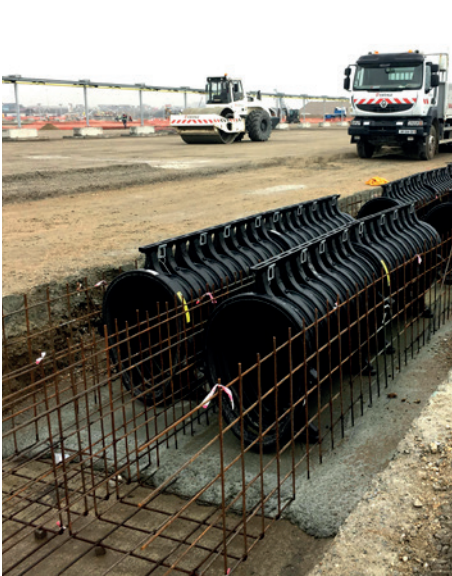
Main line installed phase 1
