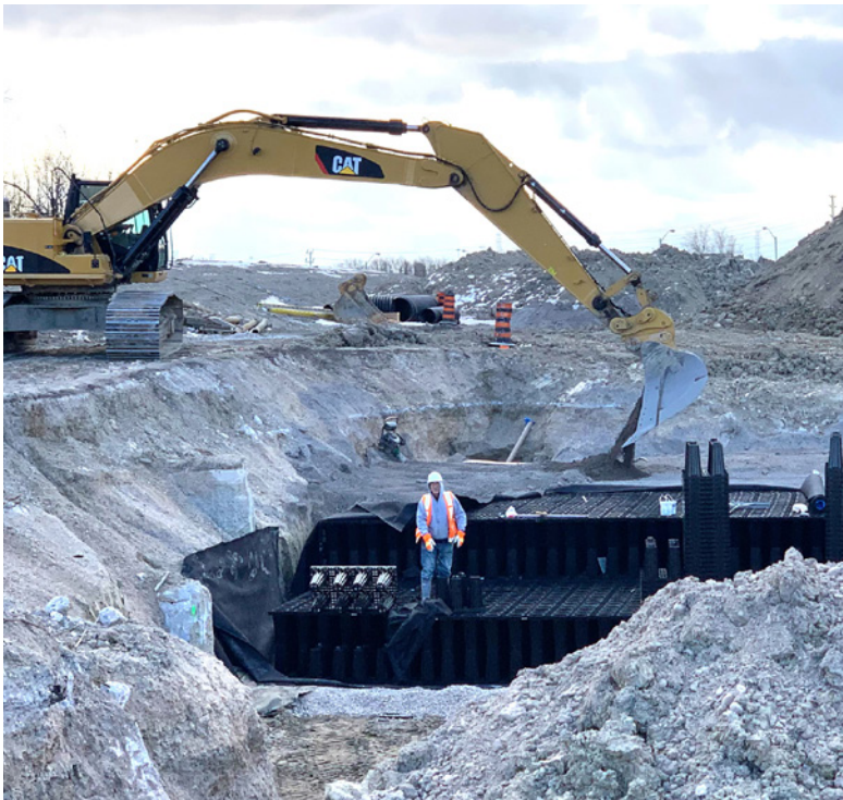
Backfilling stone on top of partially completed tank
