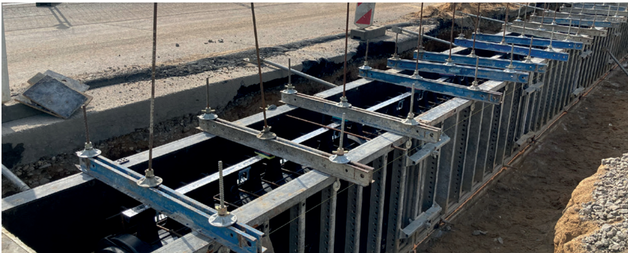
Preparation of installation site
