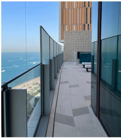
Over 13 km of stainless steel slot drainage channels are installed along the balconies
