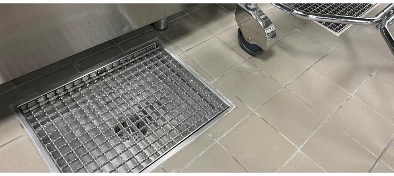
Waters in all professional kitchens are collected and treated with high quality stainless steel drainage and grease separation systems from ACO
