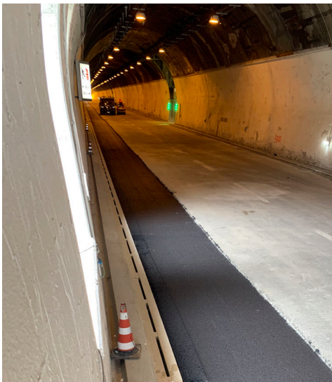
Above: ACO Monoblock S channels installed in Passo d'Avenco e Quassolo tunnels
