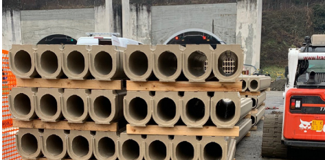
Above: stainless steel sump unit and Monoblock S channels near the Passo d'Avenco tunnel, waiting to be installed
