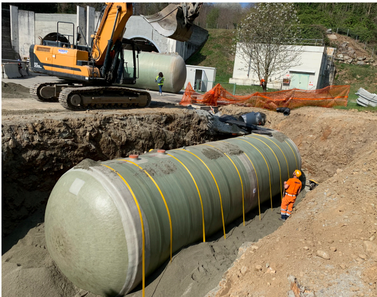
In these photos: ACO G-H tank installation phases
