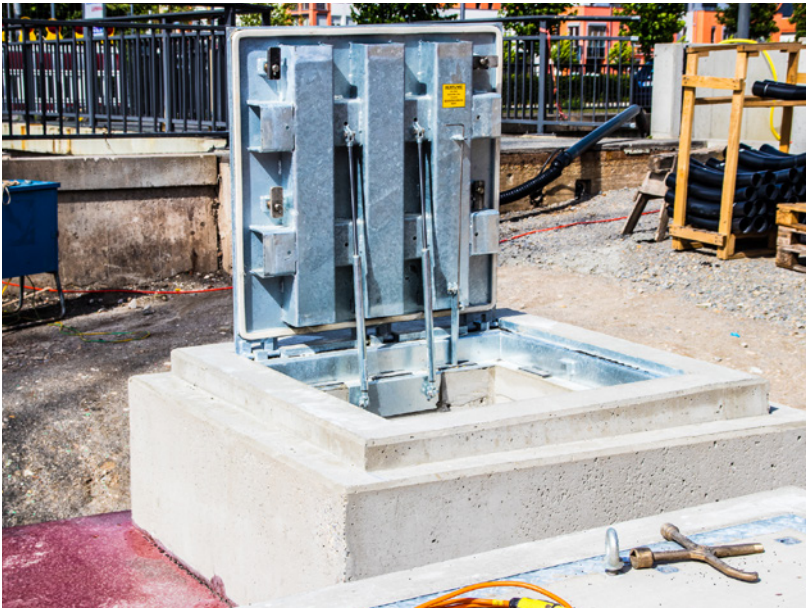
Manually actuated, backwater-proof cover with a load class of D400 and an opening aid
