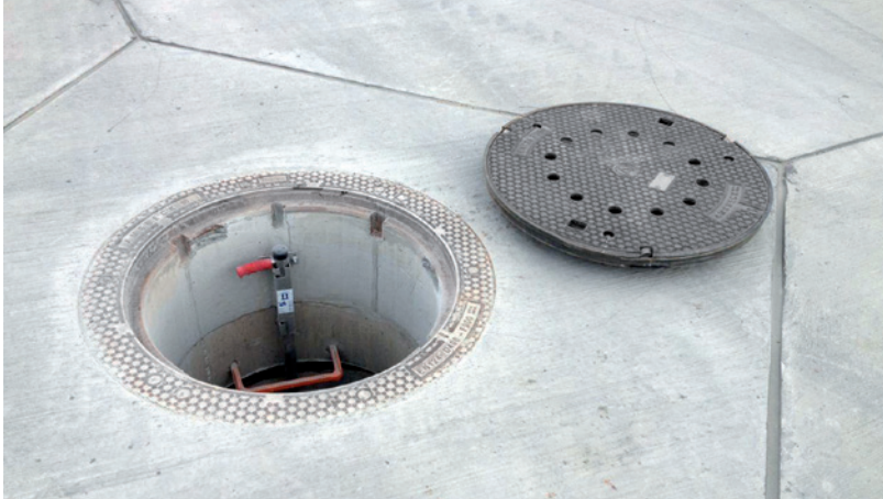
Cast-iron cover with screw-in locking lever fastenings, a load class of F900 and a clear opening of 800 mm
