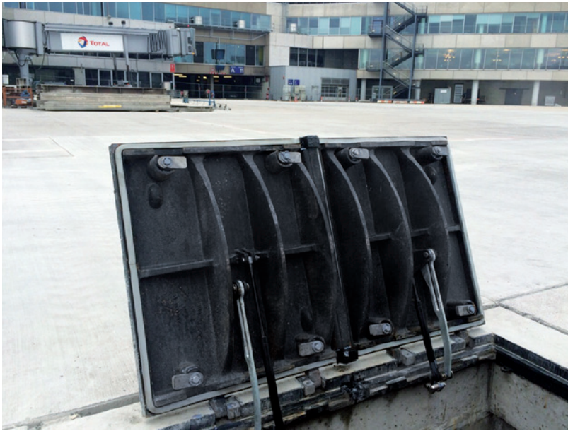
Surface-water-tight cable shaft cover with a reinforced concrete frame and a load class of F900 – Frankfurt
