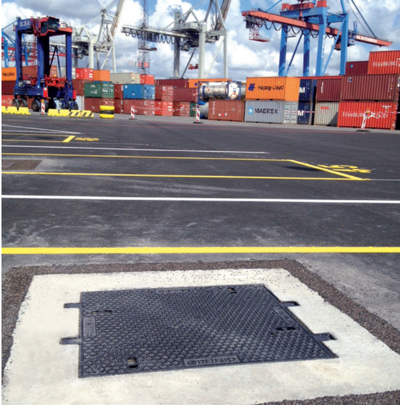
Cast-iron cover with triangular covers, a prefabricated concrete frame and a load class of F900 – Hamburg
