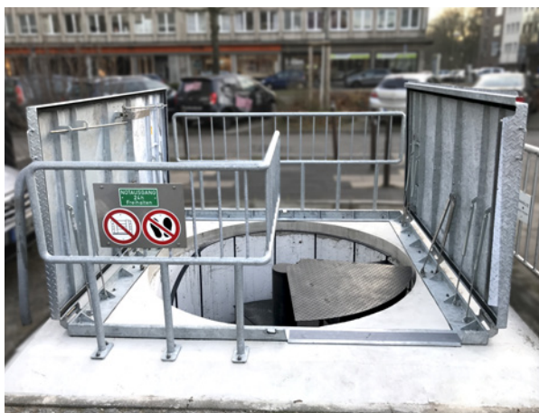
Escape hatch cover that is safe to walk on and can be operated manually – Essen
