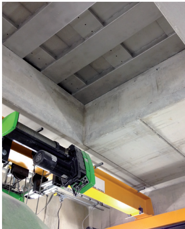
View from below of a floodproof cover on an assembly opening – power plant on the river Danube near Augsburg
