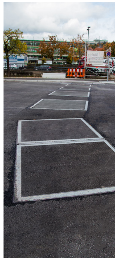
Backwater-proof covers filled with asphalt – Ansbach
