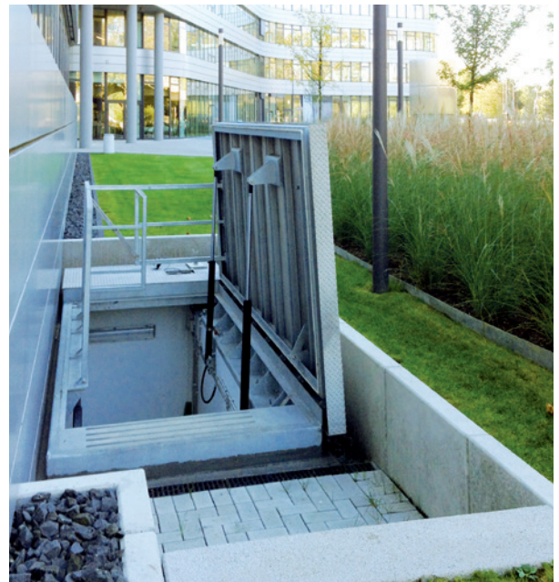
Hydraulic stainless steel escape hatch – Cologne
