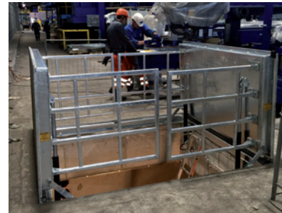
Hydraulic shaft cover as an assembly opening with anti-fall-in protection that can be driven on with a forklift truck – Krefeld
