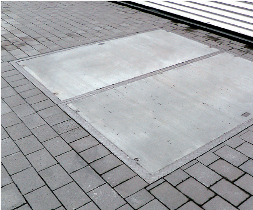
Two-piece shaft cover with concrete surface – Frankfurt
