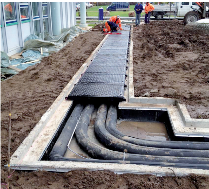
Series of cast-iron covers with a load class of B125 – Heidelberg
