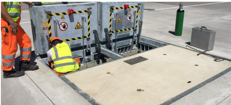
Three-piece cover with two inspection openings and a load class of F900
