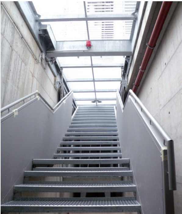
Escape hatch with a counterweight drive – Berlin
