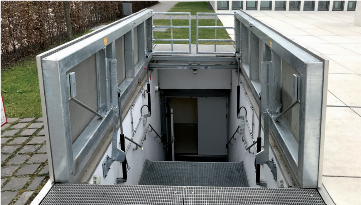
2-piece floor hatch as an emergency exit – Munich
