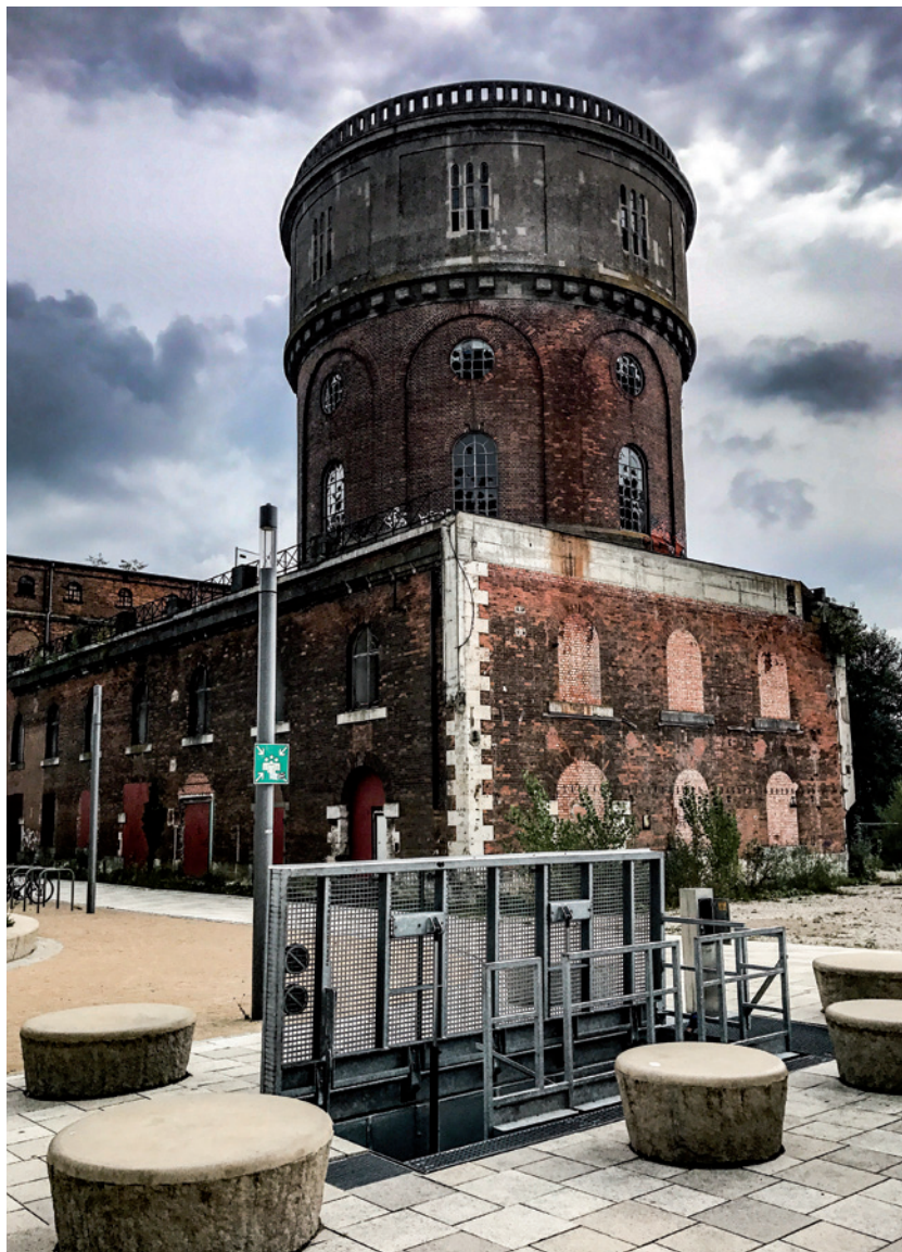
Escape hatch with a hydraulic drive and grating – Ingolstadt
