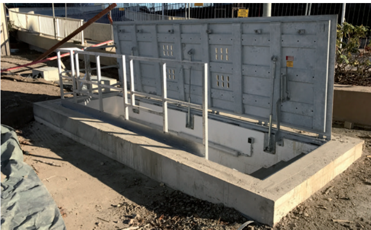
Floor hatch that can be walked on and comes equipped with an opening aid – Frankfurt
