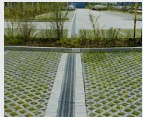
Permeable surface area coverings enable precipitation and rainwater to seep away directly from where it accumulates. During heavy rainfall and ground frost, precipitation and rainwater can be safely discharged through drainage channels
