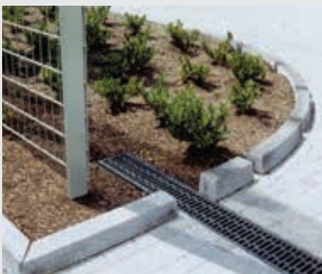
Drainage channels absorb the rainwater safely and direct it away close to the surface into the adjacent green area. There it can gradually seep away - and the plants and greenery are irrigated in a targeted manner.
