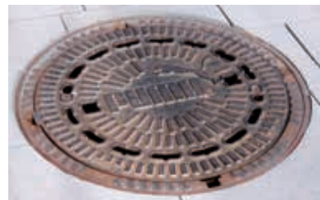
Manhole cover with company logo
