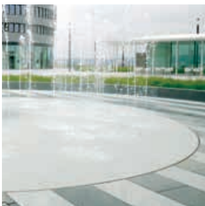
Radial slot channel
