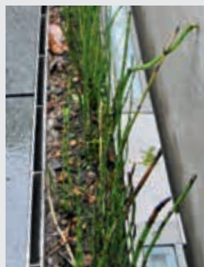
Accumulating rainwater is collected and routed to a trough near the surface
