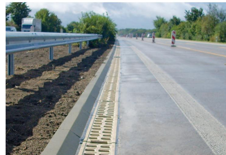
Previously: Drainage via channel + concrete kerbs
