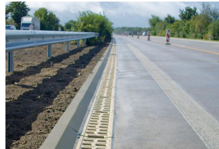
Previously: Drainage via channel + concrete kerbs
