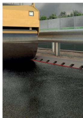
Optimal orientation for compacting machines
