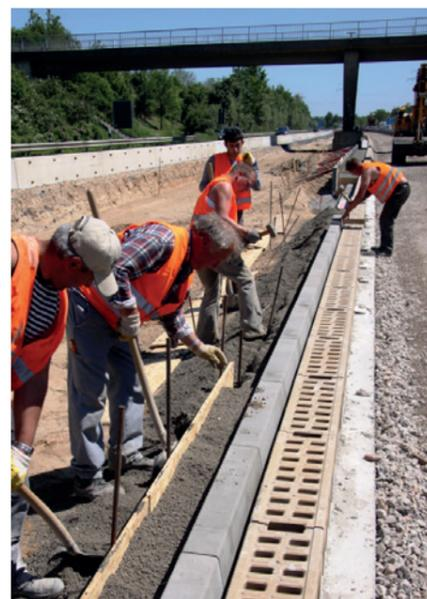
The 3-fold benefit of the new approach: the time-consuming installation of a concrete kerb is no longer necessary, the drainage is outside the road and at the same time facilitates rapid progress of construction work. In addition to the existing advantages of linear drainage of roads, as well as in combination with porous asphalt surfaces, there is a new kind of economic approach for federal traffic route construction.
