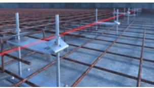
Adjusting the height of the installation aid to the desired level using a laser or cord. The height of the flange must be the same as the height of the top layer. (Lower edge of flange = top edge of background concrete) The height of the top edge of the channel (flange) must be set so that the flange does not protrude in any way, in order to ensure functional drainage. ACO channel is placed on the traverse of the ACO installation aid.
