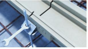
The channel is tightened with nuts (M10) at the point of contact to secure it against displacement and protrusion. This requires special care to align the channel line and transitions. The channel line should not be loaded or moved until the concrete has cured.
