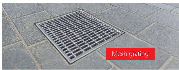
Paving stones on driveways seal the floor. A point drain allows surface water to seep away naturally.
