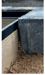
Built-in 3-5mm raised Plaster around the drain body
