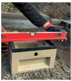
Alignment of the drain body in the concrete bedding
