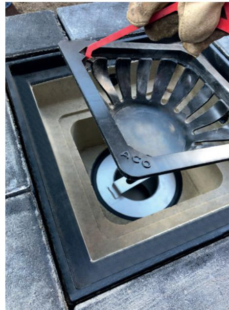
Easy handling of the silt bucket for regular cleaning
