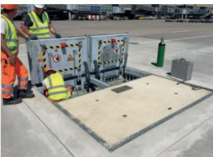
The ACO Servokat access covers are the ideal solution when covers have to be moved frequently for maintenance and inspection work. The covers with assisted-opening can be easily operated by one person. The surface covering integrated within the top is completely variable to ensure full incorporation within the design concept at each location.
