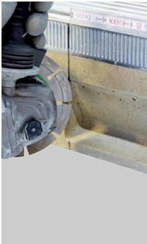
cutting the channel body to size
