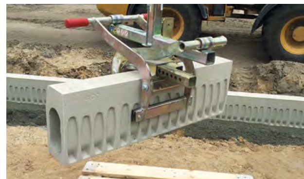
■ Pliers make it easier to move the elements
