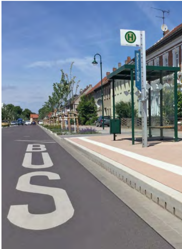
Accessible boarding of the bus thanks to the 18 cm half battered kerb
