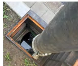
■ Rinsing the inlet chamber
