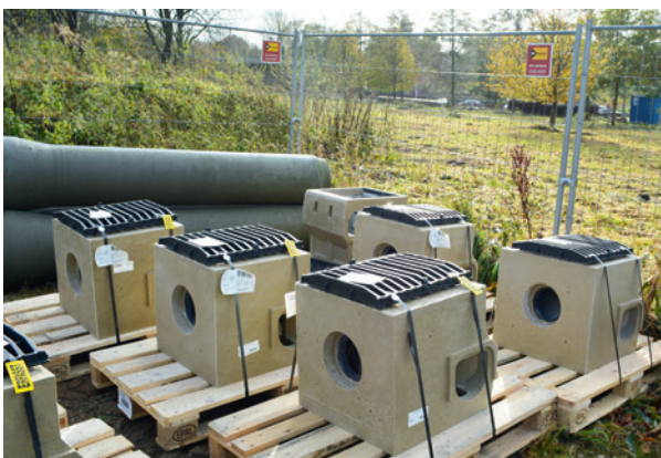
Baffle wall shafts ready to install
