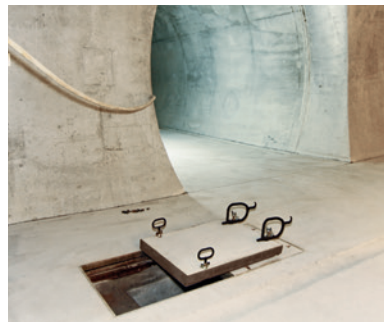
Open shaft manhole cover
