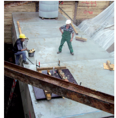
Installation example: 100,000 l fire extinguishing water tank, Mainz University, Germany
